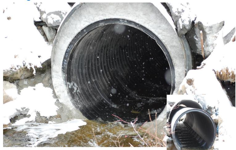
During the January cold in 2008, the City of St. John's and their contractor were busy rehabilitating a large Corrugated Steel Pipe culvert in the Goulds area. This distressed culvert showed signs of imminent failure and needed to be rehabilitated almost immediately. The City evaluated several options and concluded that Weholite pipe would be the solution for the emergency work.
